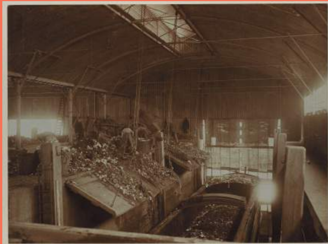
Inside a dumping shed at Nassauhaven, Men pushing waste into wasting boats.1904 16
